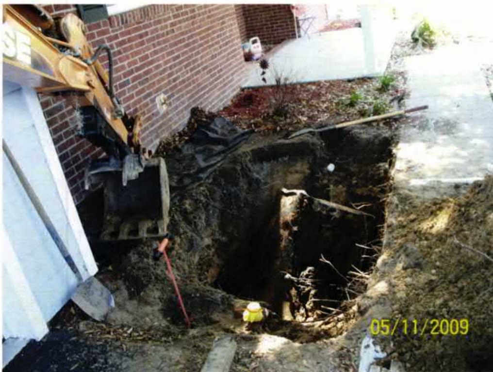
Picture 2: UST 1005Foxglove being removed from the excavation.
